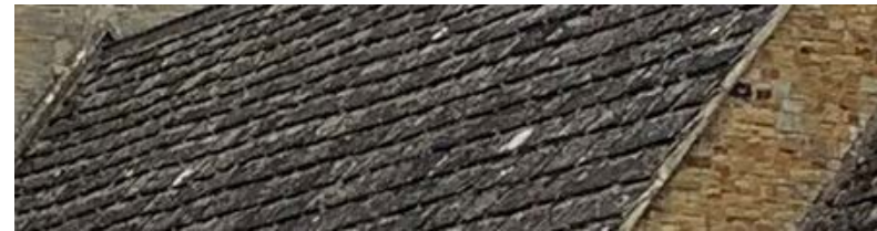
Horsham Stone slate roof
