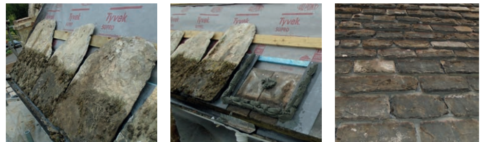
Laying of Horsham Stone slate roof with shadow slates and inconspicuous mortar
