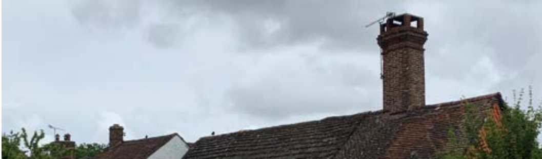
Examples of chimneys within the Conservation Area
